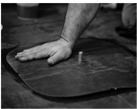
Prior to pushing the membrane down to the primed roof surface, ensure the cover membrane is aligned properly. Once properly aligned, pressed down firmly to the roof surface with your hands to adhere the primed EPDM surface without any wrinkles or air pockets.
