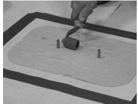
Repeat with the remaining half of the fabric over the bolt, pressing it down firmly. Roll with a 2-inch roller to properly adhere the fabric to the roof surface.
