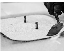
Using a trowel and propane torch, lift the membrane and apply heat to seal leaving a 1/4 **inch bleed out** around the perimeter of the cover membrane.
