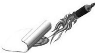
**Step 1:** Once properly aligned, outline the target area and remove the target. Apply heat to the substrate to embed granules into the membrane with a trowel. Secure the plate with approved fasteners, per engineering requirements.
